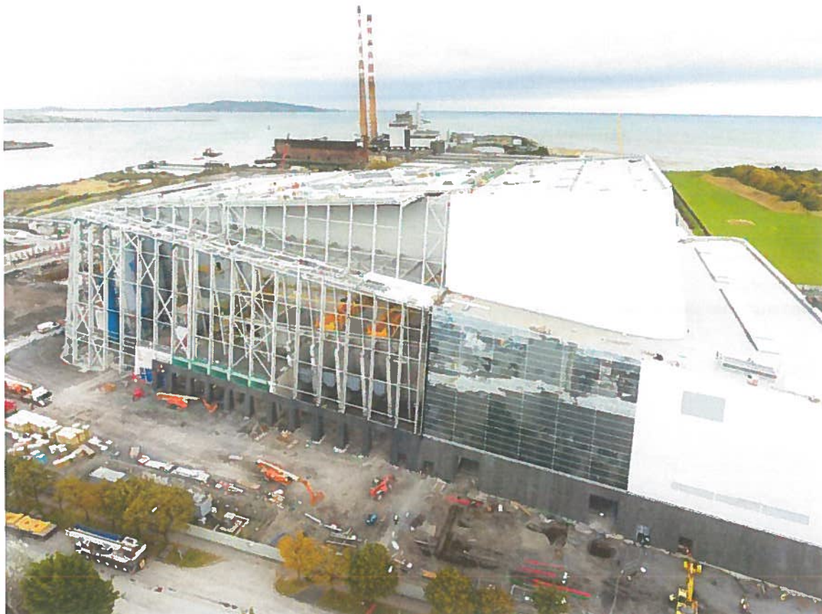
Site Aerial view looking East October 2016 (Copyright PML)
